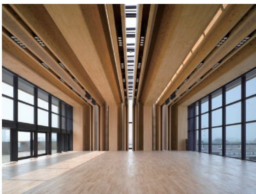
Hall on top floor. Wooden beams span approximately 30m.
