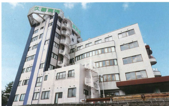
External appearance of Building
