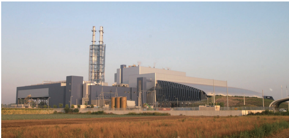
Photograph of Facility (Naples, Italy)(Source: Steinmüller Babcock Environment GmbH)
