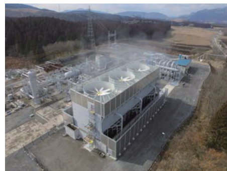
Takigami binary power plant (Japan) Output: 5.05 MW In operation since 2017
