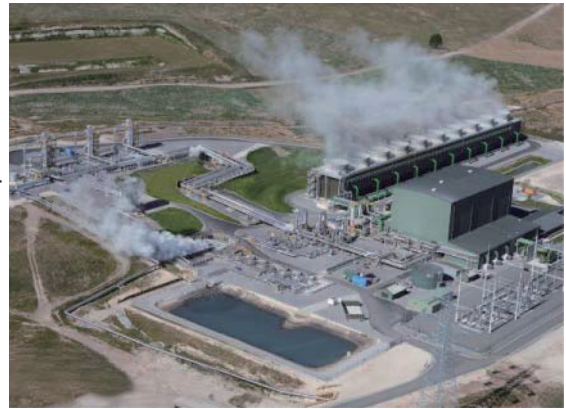
Nga Awa Purua geothermal power plant (New Zealand) In operation since 2010
