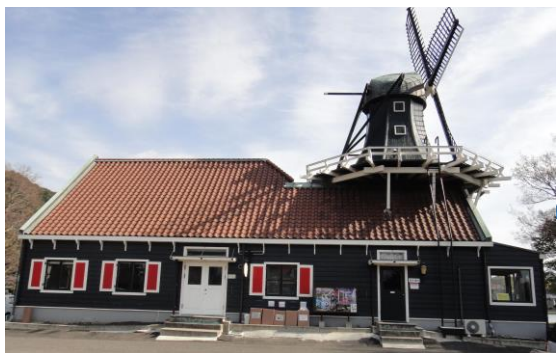
Administrative Building (Lighting & Air Conditioner)
